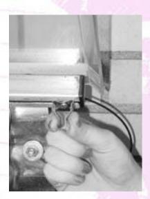
3. Attach the safety retainer-hinge lanyards to the top bolts that mount the areawall to the foundation. \*Alternatively, anchor the loop end of the lanyard to the home foundation or directly to the areawall itself, depending on your particular application. Allow for enough lanyard length so the cover will pivot up and stay propped open against the side of the house.
